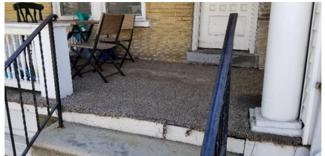
Porch Floor Decking (Applicant)
