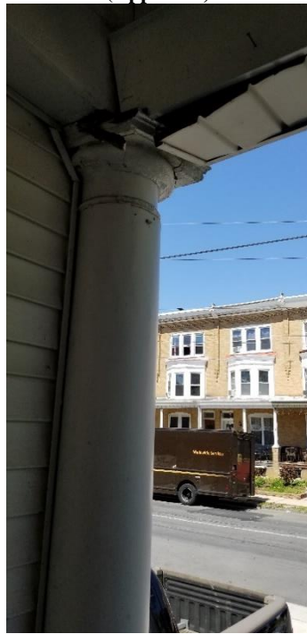
Porch Column and Header (Applicant)
