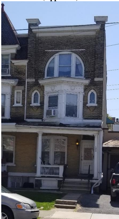
Primary Façade, view looking south (Applicant)
