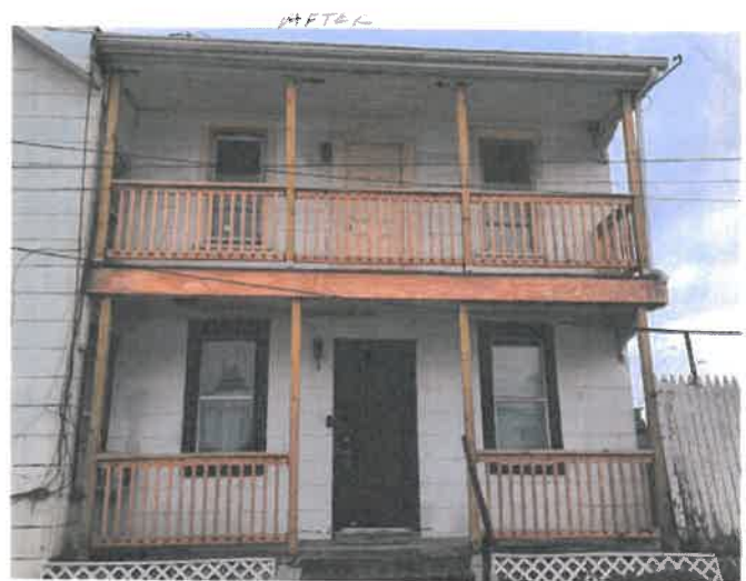
Law Street elevation of 526 Liberty Street after work was completed. (Staff)
