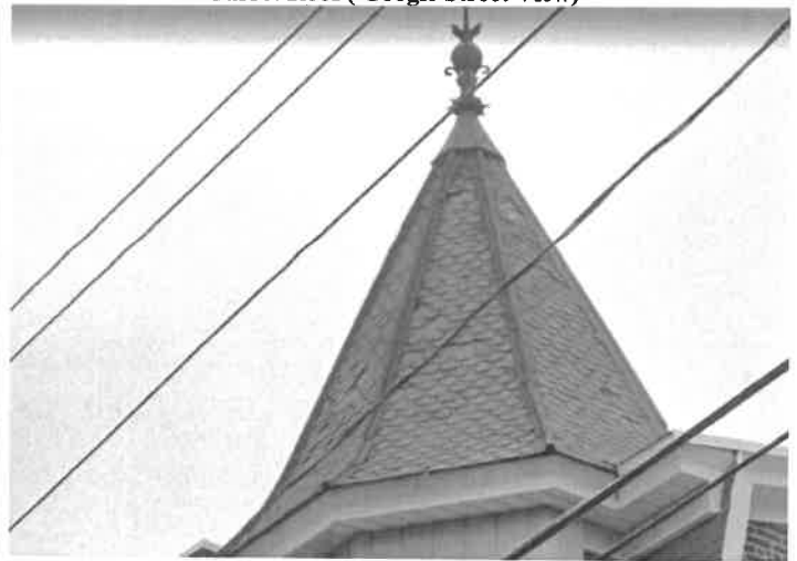
Turret Roof ( Google Street View)
