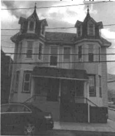
Primary Façade (Applicant)
