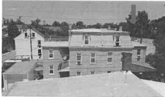
Primary Facade from Neighboring Building, 1015 Oak St. indicated with arrow (Applicant)
