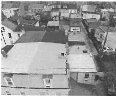
Aerial of Roof (Applicant)
