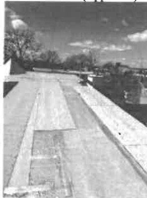
3 rd Floor Roof (Applicant)
