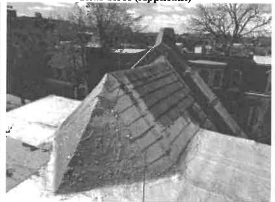
Rear Roof (Applicant)
