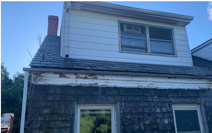
Existing rear slate roof at 433 N. 11th Street. (Applicant)
