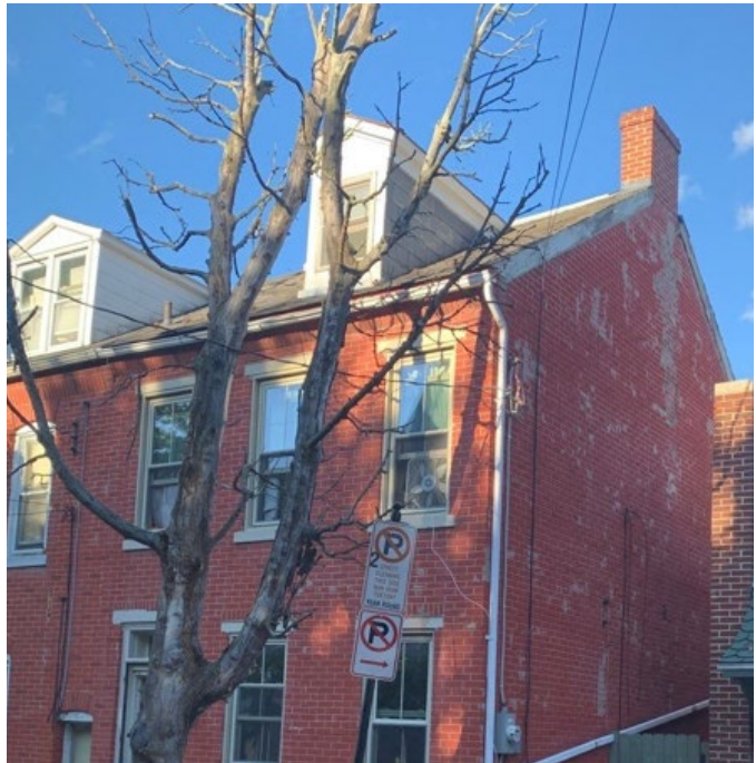
Existing slate roof at 433 N. 11th Street. (Applicant)
