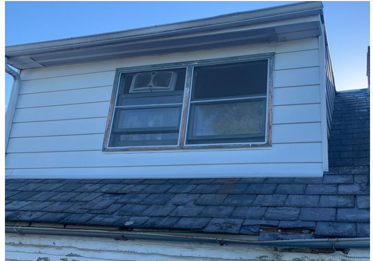
Existing rear slate roof at 433 N. 11th Street. (Applicant)
