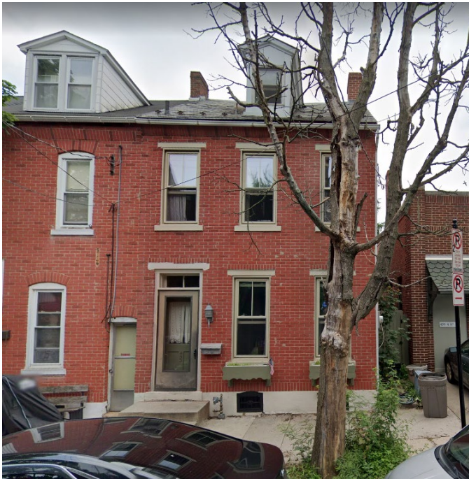
Existing slate roof at 433 N. 11th Street, 2019. (Google StreetView)
