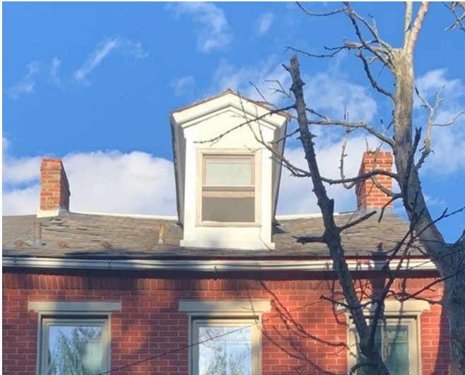
Existing slate roof at 433 N. 11th Street. (Applicant)
