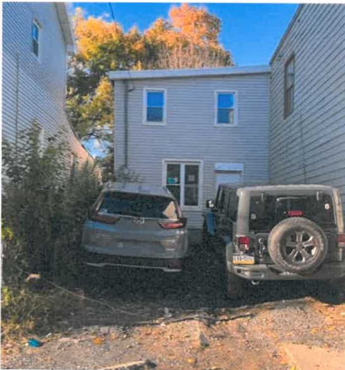
933 W. Pine Street after exterior alterations. (Applicant)
