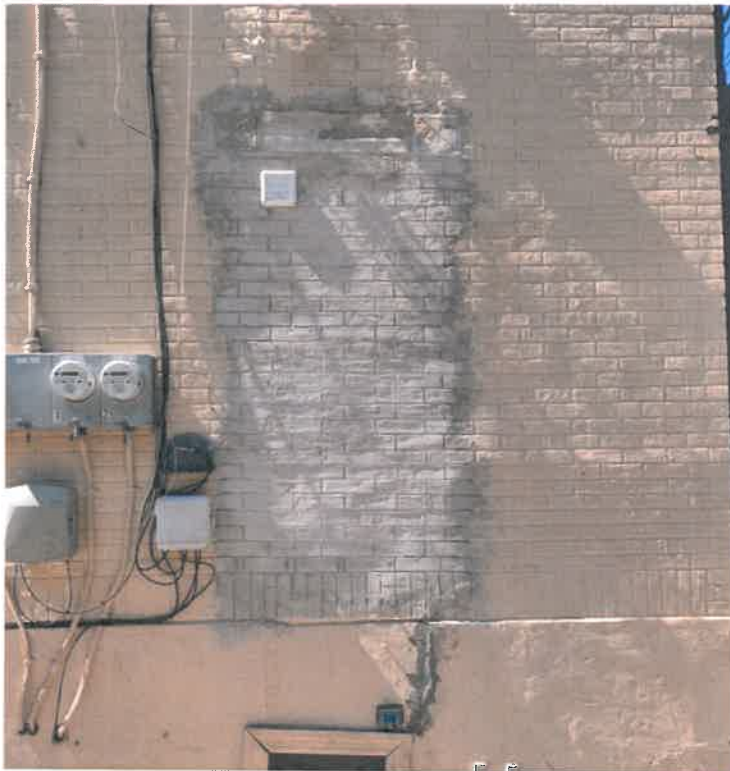
Refwal Street window after being infilled. (Applicant)
