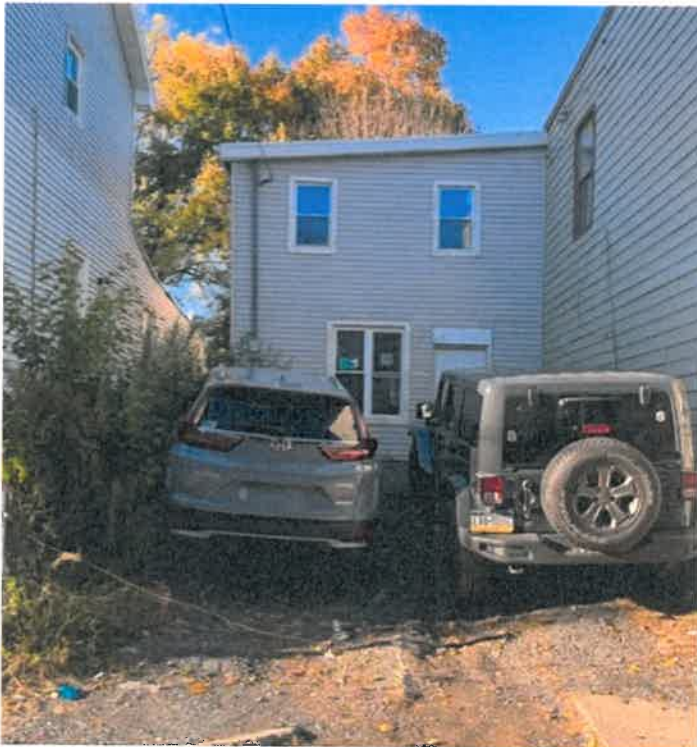
933 W. Pine Street after exterior alterations. (Applicant)
