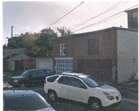
One- and two-story garages in the immediate vicinity. (Google StreetView)
