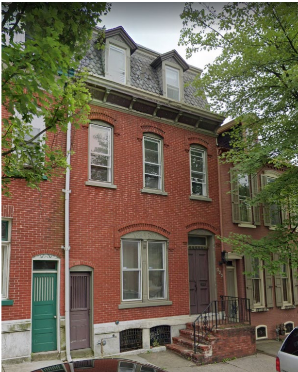
Front façade of 322 N. 8 th Street, 2019. (Google)
